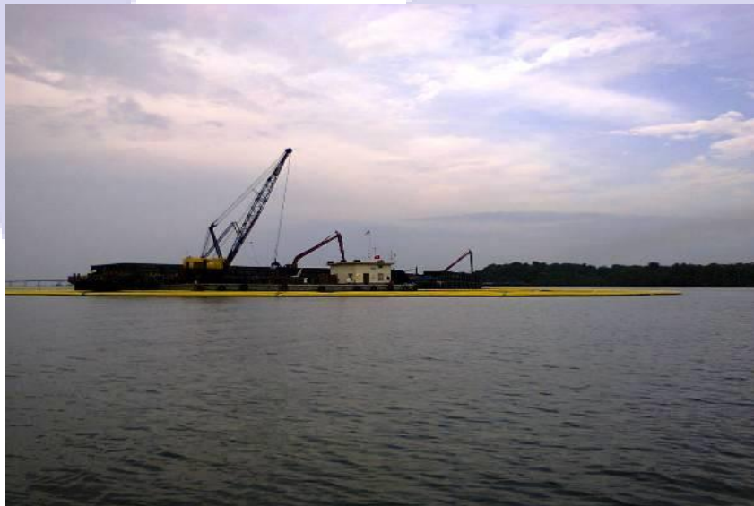
Installation of double layer silt curtain
