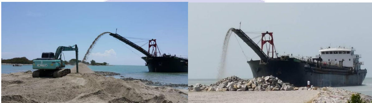
Delivery of marine sand using trailing 3 in 1 suction hopper.
