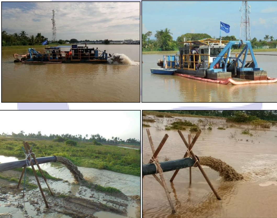
Performance of Maintenance Dredging Works within “Balancing Pond, Sungai Dua, Pulau Pinang, Perbadanan Bekalan Air Pulau Pinang (PBAPP)”
